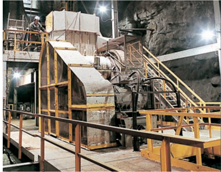
C160 at an underground gold mine.
