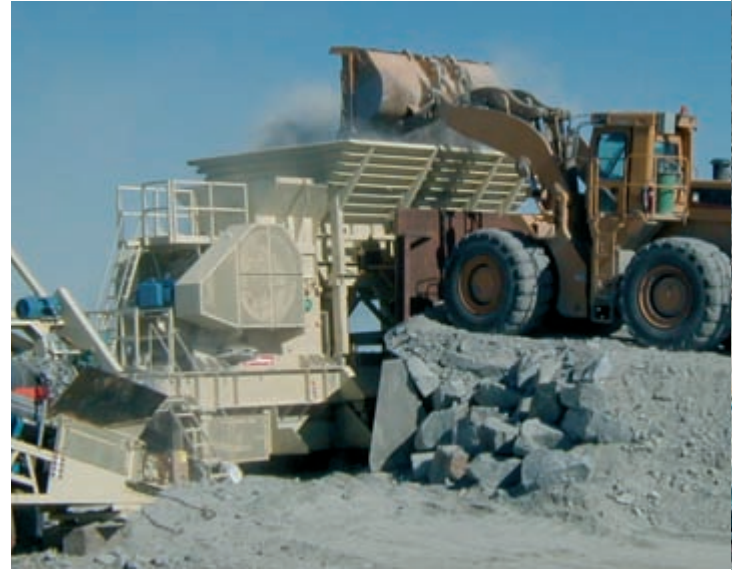
Mobile crushing with the NW125.
