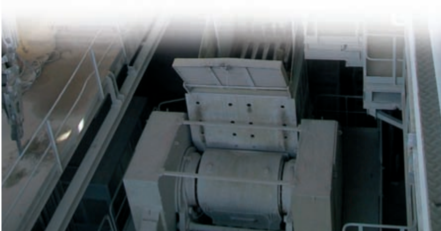
A C200 after replacement of a double toggle jaw crusher. Plant capacity was increased without having to modify the foundations.
